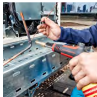
Brazing in refrigeration / air-conditioning technology
