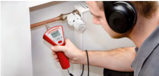
Acoustic leak detection of heating installations
