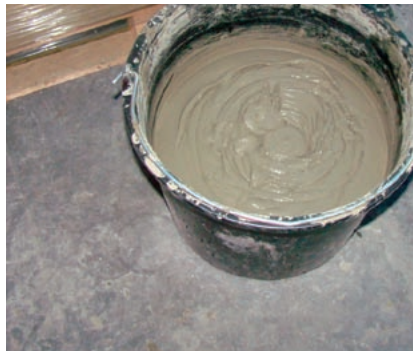
Prepare Dexaflamm B cement
