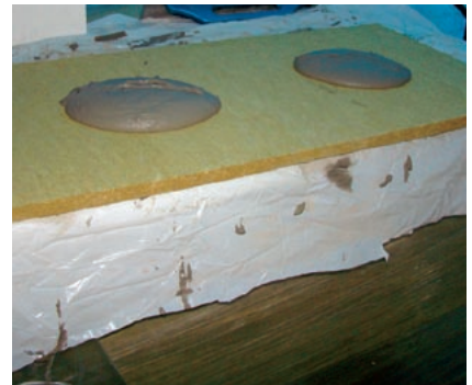
Apply an adequate amount of the cement on the slab
