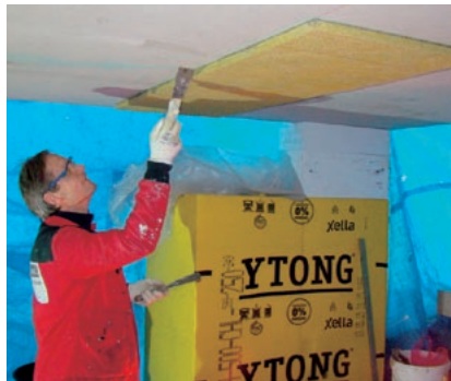
Press the first slab to the baseline and remove any excessive glue
