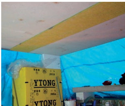
Installation of the first row of slabs - inspect the straightness of the row
