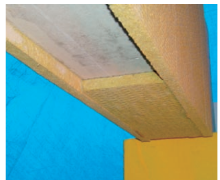
The flange is glued in the end
