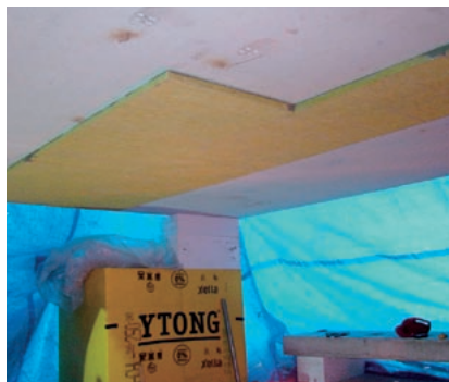
Install other slabs by pressing them against the edge of the already installed slabs (the edges are not glued)
