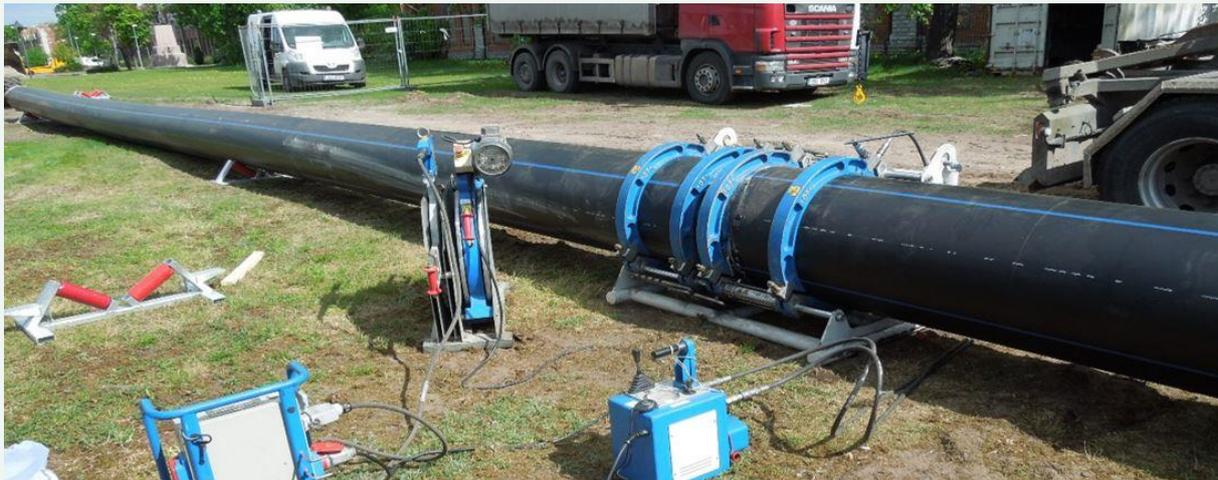
**Figure 1.** HDPE pressure pipes installation process stage
