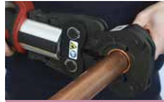
3. Complete the joint with the press tool
