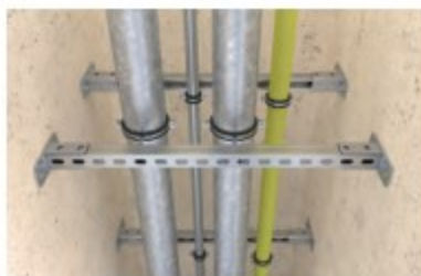
Pipe installation in escape route
