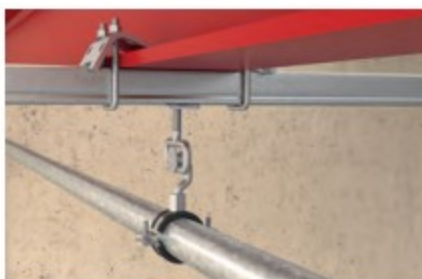
Channel to steelbeam
