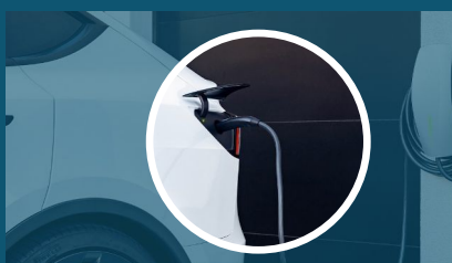
Electric Vehicle Charging Outlet in Garage & 200 AMP Service
