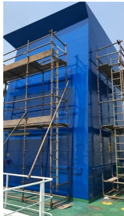
SCAFFOLDING ERECTED FOR PAINTING OF COMPANY LOGO ON FUNNEL
