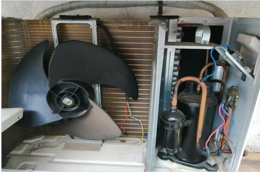
Fig. 2.2: Unitary Air Conditioner (Actual Image)
