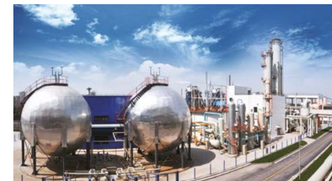
Credit: Shanghai Shidongkou Coal-Fired Power CO 2 Capture Facility, image courtesy of Huaneng Clean Energy Research Institute.
