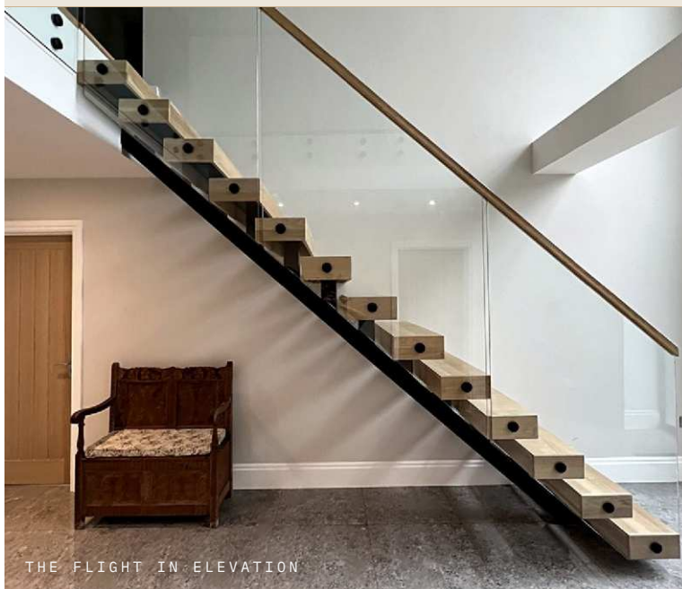
TREAD ENDS &amp; STANDOFF FIXINGS
