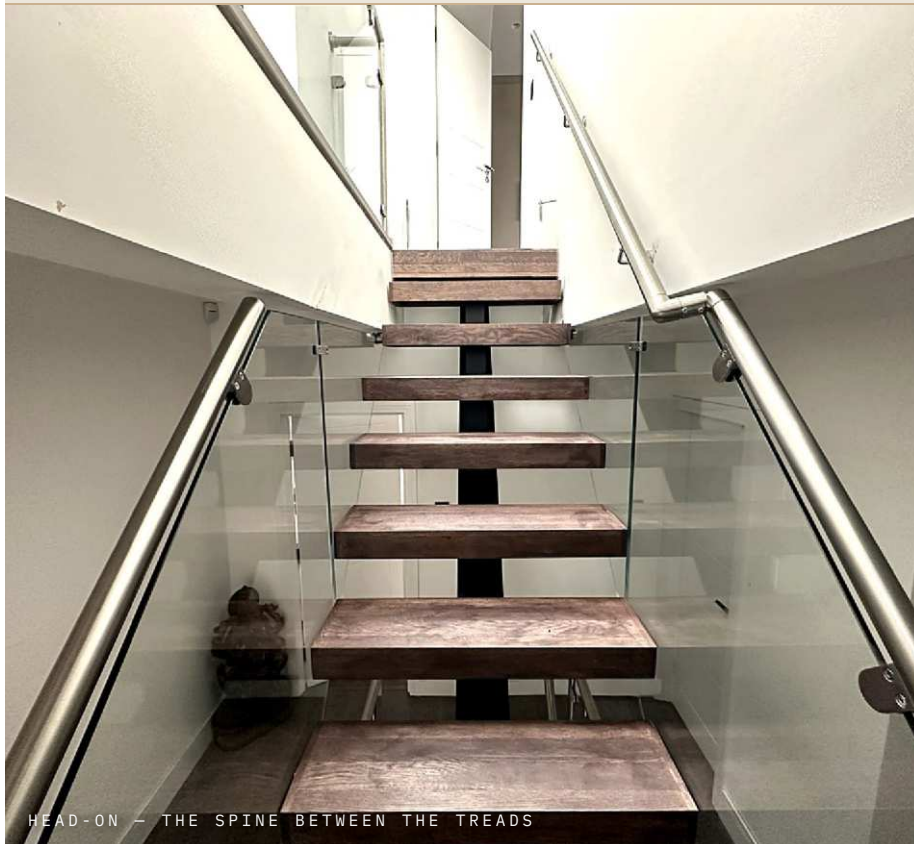
TREADS &amp; STANDOFF FIXINGS
