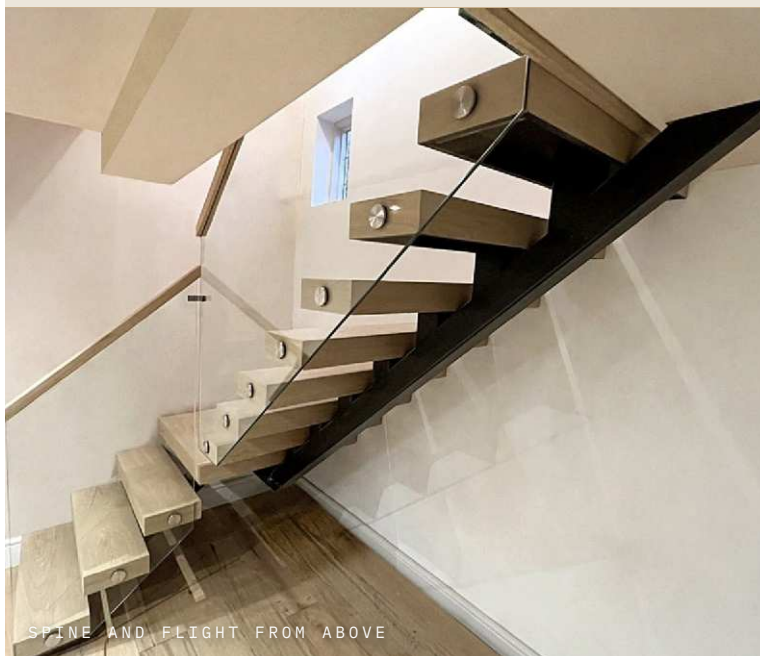
SPLOYED TREADS AT THE FOOT
