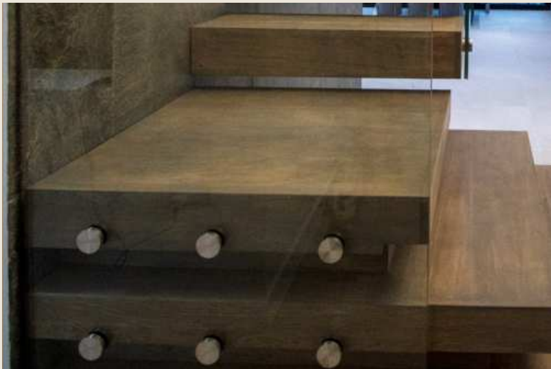
DETAIL — PYRAMID BASE & STANDOFF-FIXED GLASS
