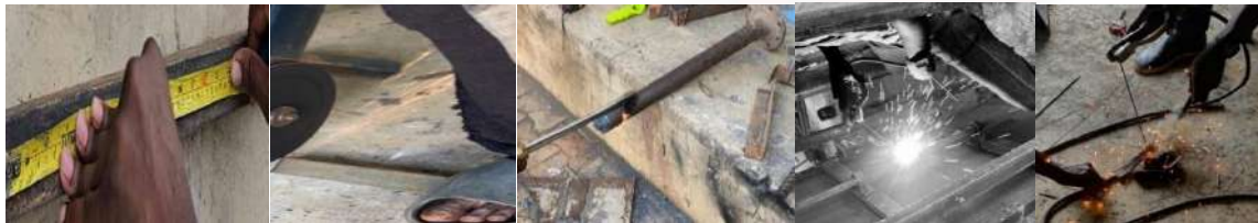
a. Marking out b. Cutting using an angle grinder c. Cutting using a gas blow torch d. Welding process
