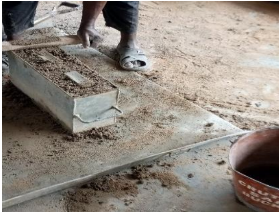
Figure 2: Manual moulding of sandcrete block
