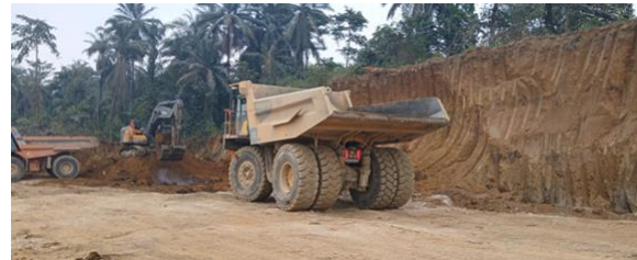
FIGURE 1: OVERBURDEN BEING STRIPPED TO EXPOSE LIMESTONE
