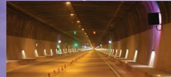
2017 Chenani - Nashri Tunnel, Jammu & Kashmir
