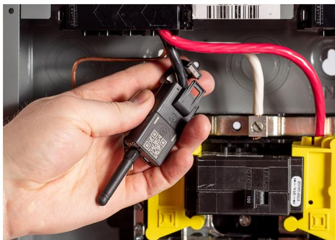
The Core can detach from the HotDrop CT for larger CT sizes
