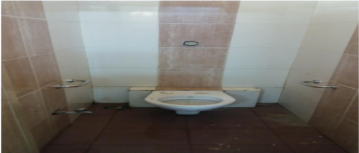
Wash Room (Boys )
