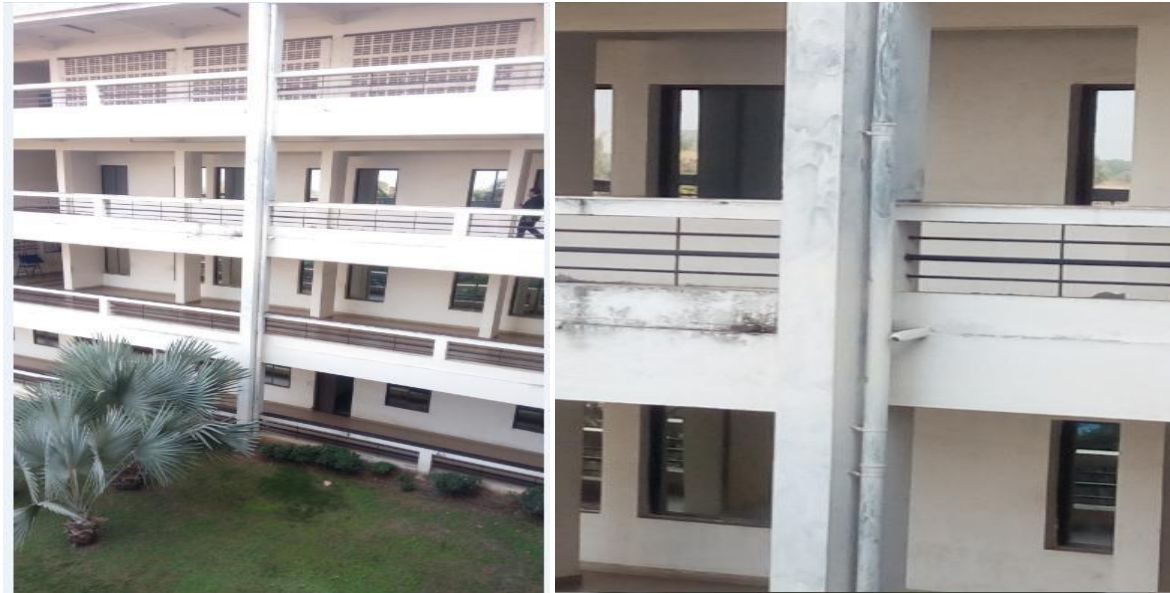
7.1.4.1 Rain water harvesting at B-Block building
