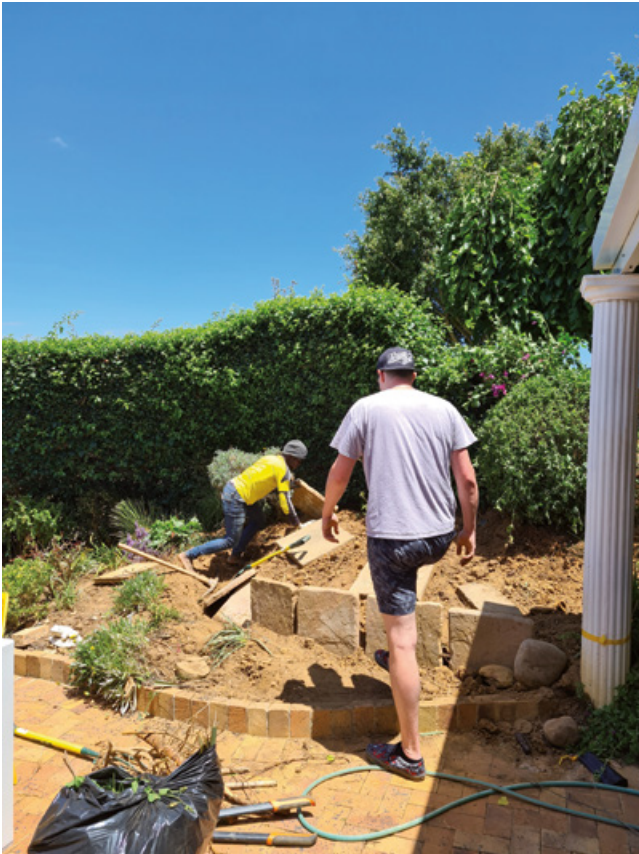
BEFORE: Laying out the Garden terrasses
