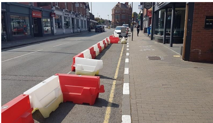
Temporary barriers – maintenance issues
