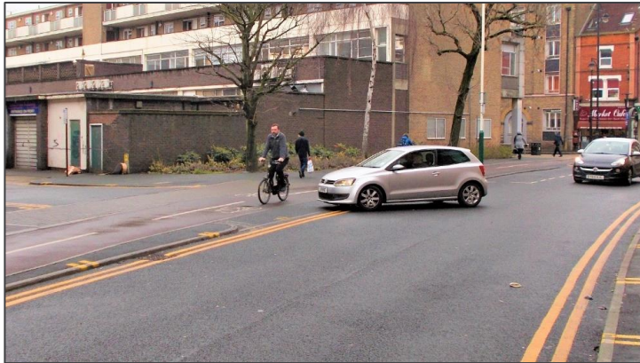
Continuous footway & cycle track.
