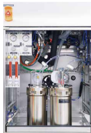
Cabinet with CPDs and flow meters
