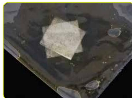
3. Wet the StickNET fibres with resin
