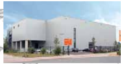
MEISINGER Germany Headquarters, Neuss
