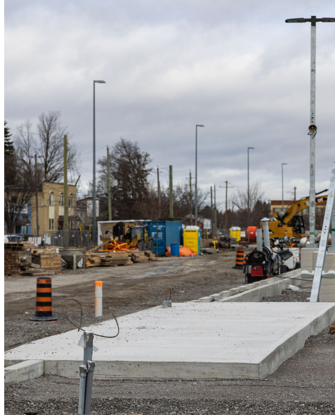
A shelter pad on the new west platform. Metrolinx image
