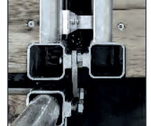
Place the Junction Plate inward if it's the end dock section.
