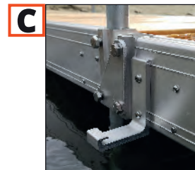
Place the Junction Plate inward if it's the end dock section.
