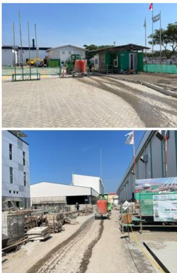
Dust Control by Water Spraying
