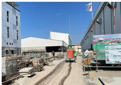
Dust control program by water spraying
