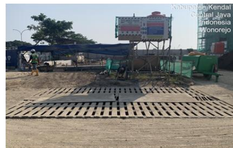
Washing bay for washing vehicle wheels before leaving the project
