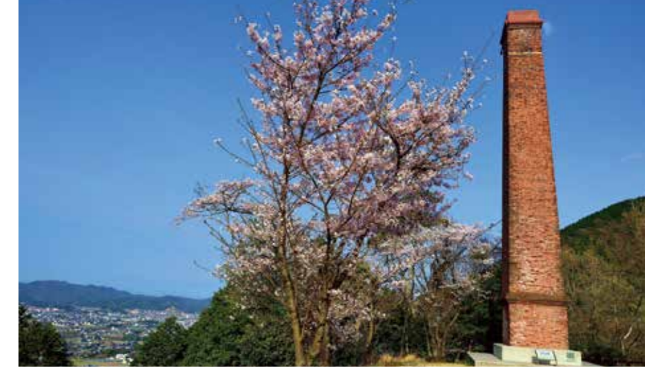
Chimney of former Yamane Refinery
