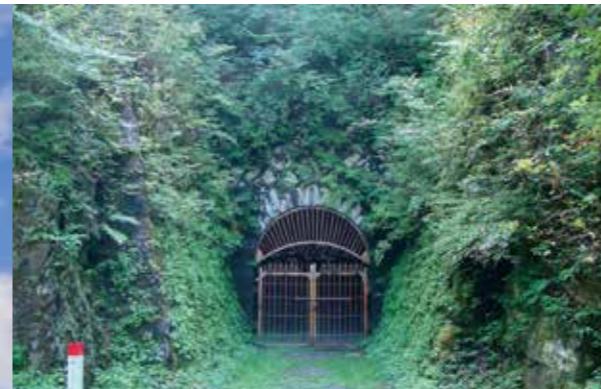
The No.3 Main Tunnel
