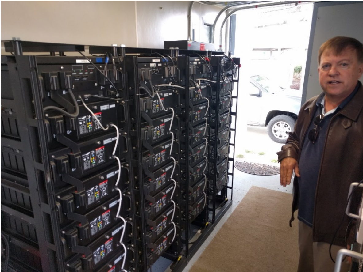
Frank Bishop of Gridscape Solutions demonstrates the internal batteries and controls of the Fremont Fire Station Microgrid
