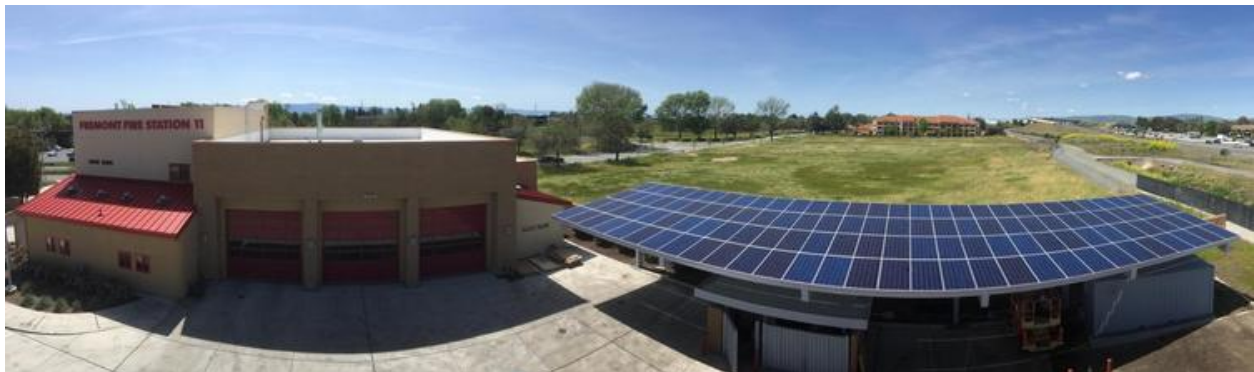
Fremont Fire Station 11 Microgrid, a model for emergency services microgrids developed by Gridscope Solutions
