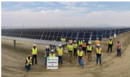
Rosamond Central Solar Project
