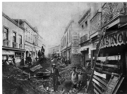
Figure 6. Photographic Evidence of Collapsed Informal Housing in Valparaíso, 1906 Earthquake
