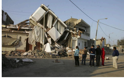
Figure 7. Post-Earthquake Building Conditions in Pisco, 2007.
