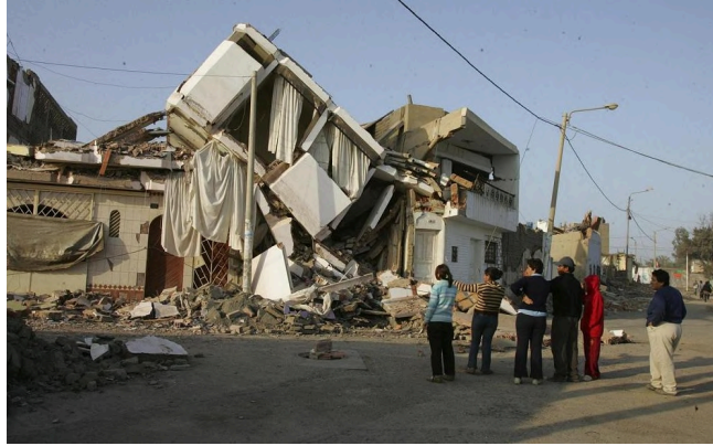
Figure 5: Post-Earthquake Building Conditions in Pisco, 2007.
