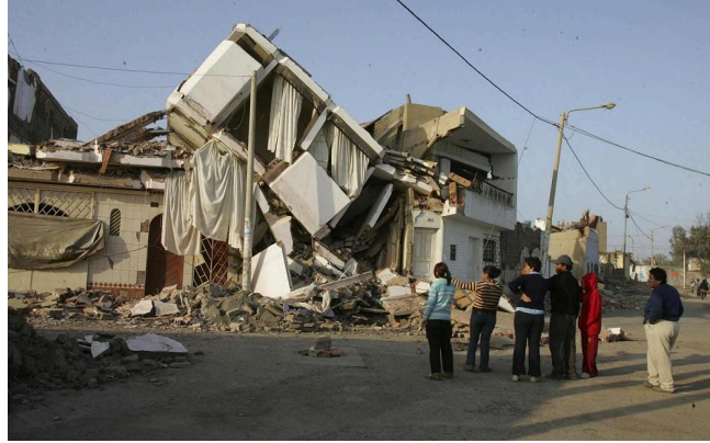
Figure 5: Post-Earthquake Building Conditions in Pisco, 2007.
