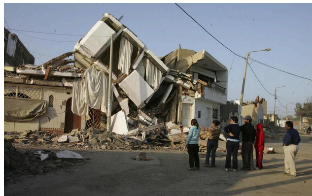
Figure 5: Post-Earthquake Building Conditions in Pisco, 2007.
