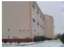
Fort Knox potable water corrosion prevention
