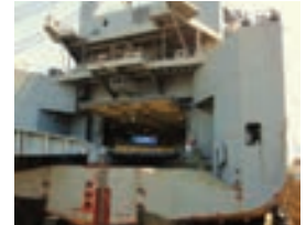
USNS Watkins venting pipes, air and oil
