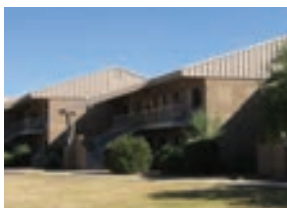
Davis AFB pinhole leaks copper
