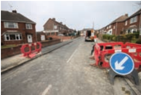
Lead Service Lines - No Road Closure
