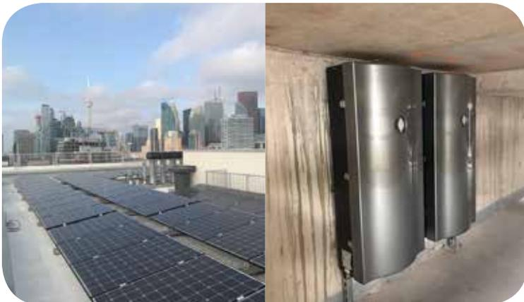
Tridel, Canada's largest builder of sustainable condominiums, integrated the IQ System with rooftop solar panels for the penthouse suite of the new Aqualina complex in Toronto. Installed in August 2017, the system is designed to maximize the owner's ability to self-consume solar and provide a solar+storage microgrid for backup power when the grid goes down.
