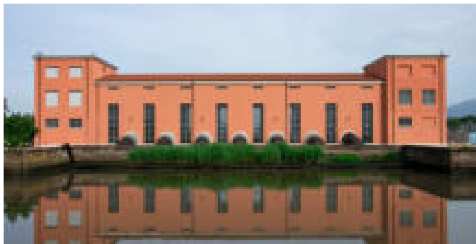
I. Pontinia, Mazzocchio pumping station. Photo courtesy of the Lazio South West Land Reclamation Consortium.
