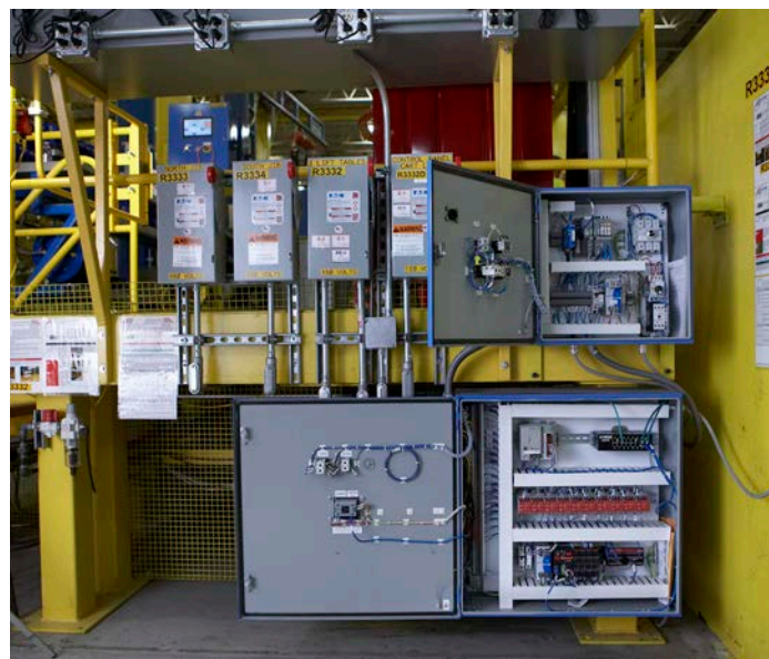
Figure 7.6.5.a Existing installation labeling per 240.86(A) and 110.22(B).
