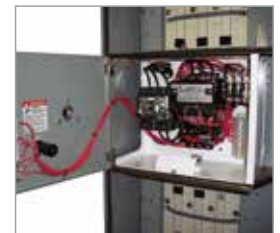
Square D replacement MCC unit installed in General Electric 7700 Series structure
