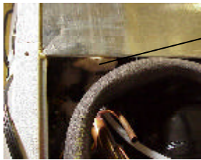
Using the permagum provided in kit, seal hole and end of old heat exchanger.
