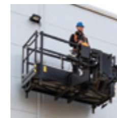
Man platform ready
