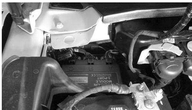
Isolation module, after installation.
