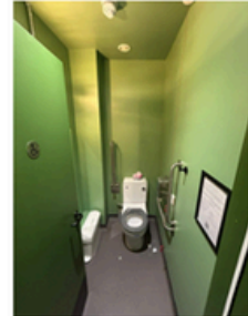
Disabled cubicle (Support rail, emergency cord)
