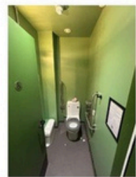
Toilet with Support rail and emergency cord
