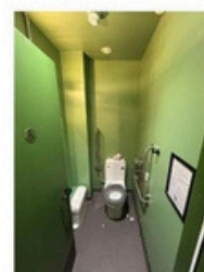
Toilet with Support rail and emergency cord
