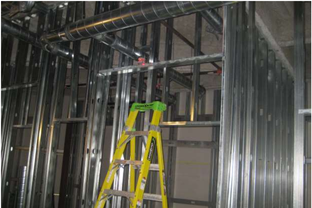
Photo 2382 – View of missing metal stud framing at the third floor. To be repaired by DC worker, Trevor.
