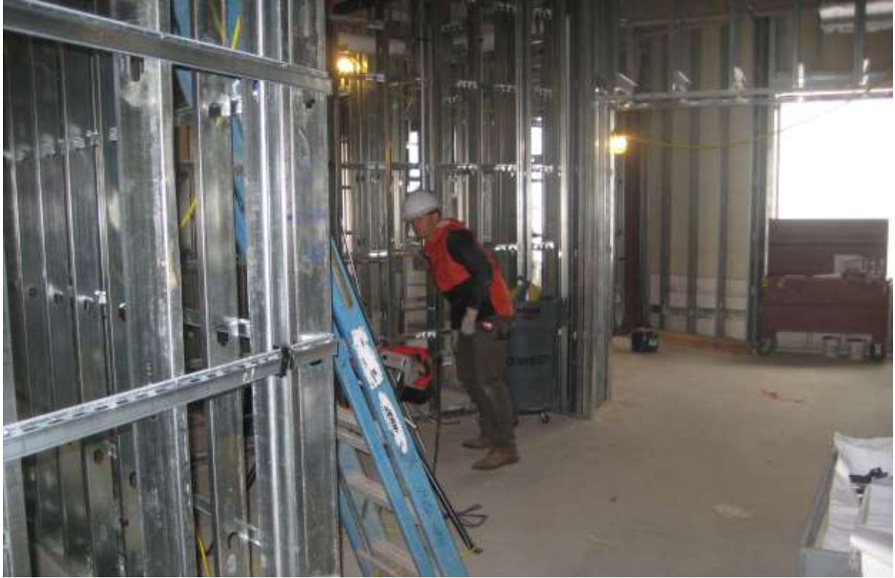
Photo 2381 – EE worker, Brian, installs electrical conduit into wall cavities at the second floor level.
