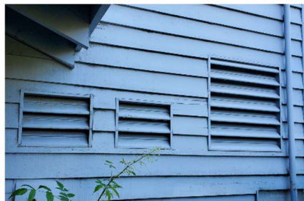
Boiler room relief and outside air louver
