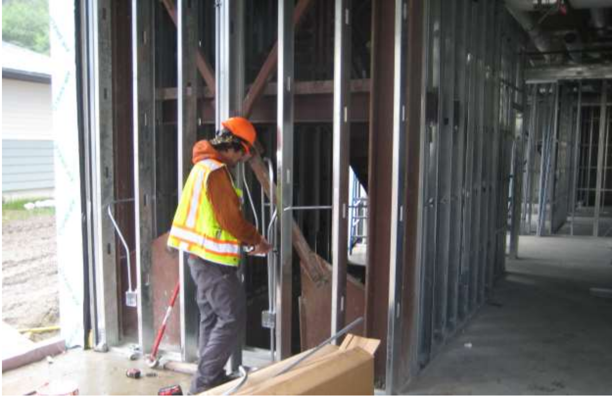
Photo 2379 – EE worker, Robert, installs electrical conduit into wall cavities at the first floor level.
