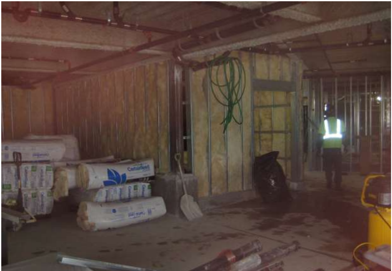
Photo 2376 – DC's two-man work crew, Gregg and Riley, installs batt insulation at interior, partition walls at the basement level.
