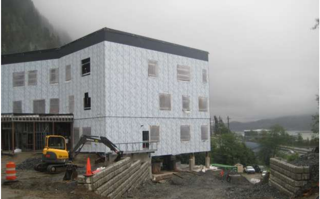
Photo 2375 – View of west façade, where DC workers, have completed the wind/vapor barrier installation.
