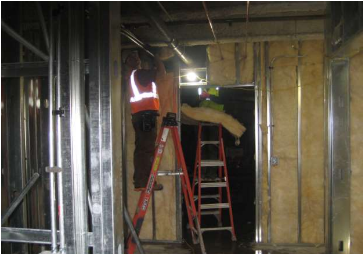
Photo 2378 – Continuation of wall insulation (by Gregg) at the basement level. Note presence of Long Control's worker, Adam, shown (in foreground) installing HVAC control (wiring) conduits.
