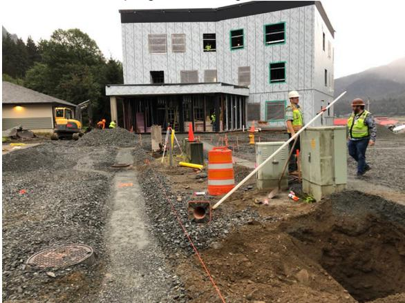
3. Photo 8618: SEEM at work prepping drive and concrete walk area at building entry.
