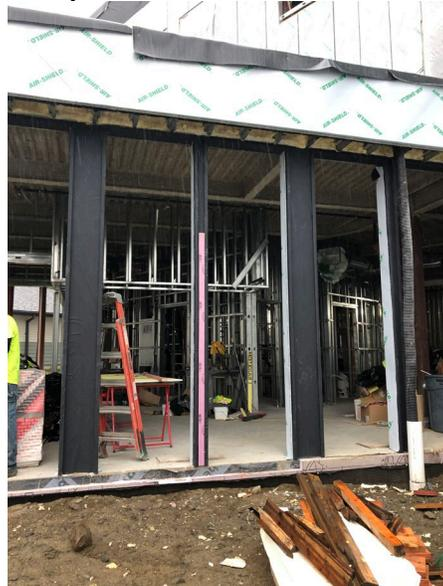
6. Photo 8620: DC worker installing air-shield at interior face of storefront framing.
