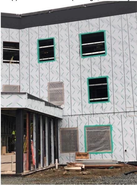
9. Photo 8626: DC worker installing 5/8" plywood backing and window rough openings.
