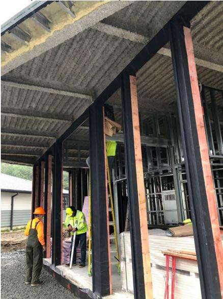
5. Photo 8629 – DC installing insulation and WRB-1 at exterior face of storefront framing at entry.
