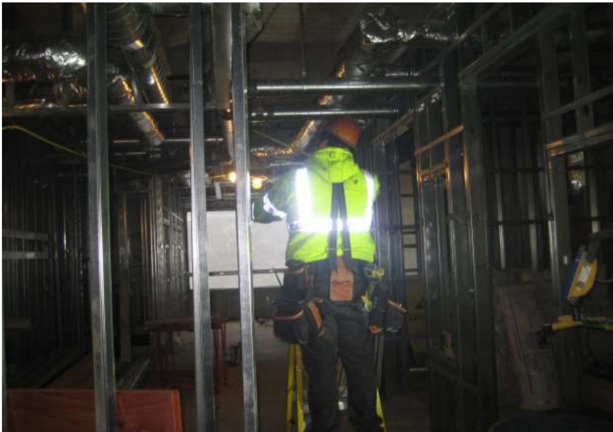
Photo 2681 – DC worker, Trevor, prepares to install pocket sliding doorway header crossing corridor 322-E near room 310 EAST, Patient Room , at third floor level.
