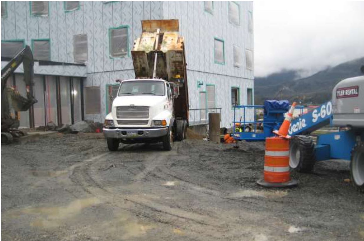
Photo 2689 – SEEM owner, Jon McGraw, delivers fill materials to the upper parking area for use in backfilling the new retaining wall. Note large boulders at planting bed in background.
