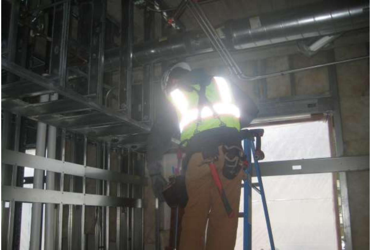
Photo 2683 – EE worker, Brian (apprentice), shown installing electrical components into the ceiling cavity of room 226, Break Room , second floor level.
