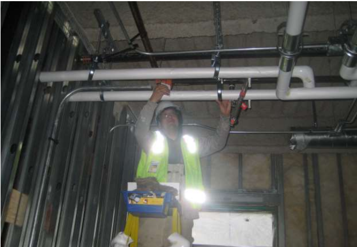
Photo 2680 – AIS worker, Tom, installs rigid glass pipe insulation to copper supply lines on the third floor in room 315, Break Room .
