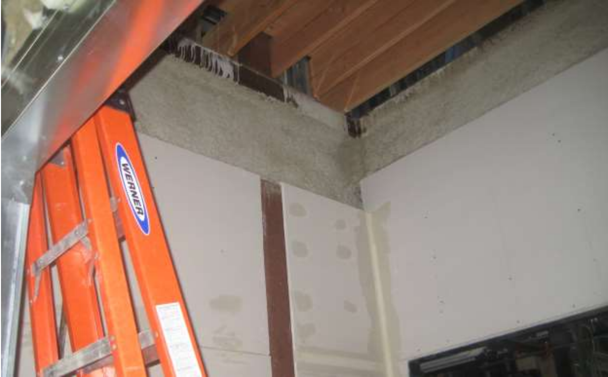
Photo 2685 – CC’s drywall workforce, Mike and Jose, ‘tape and mud’ final layer of 5/8” GWB sheetrock wall surfaces at the elevator shaft way, second floor.
