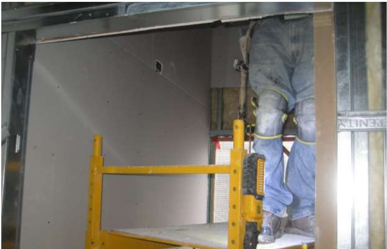
Photo 2684 – – CC's drywall workforce, consisting of two laborers, installs first layer of 5/8" GWB sheetrock within the northwest stairway, first floor level.
