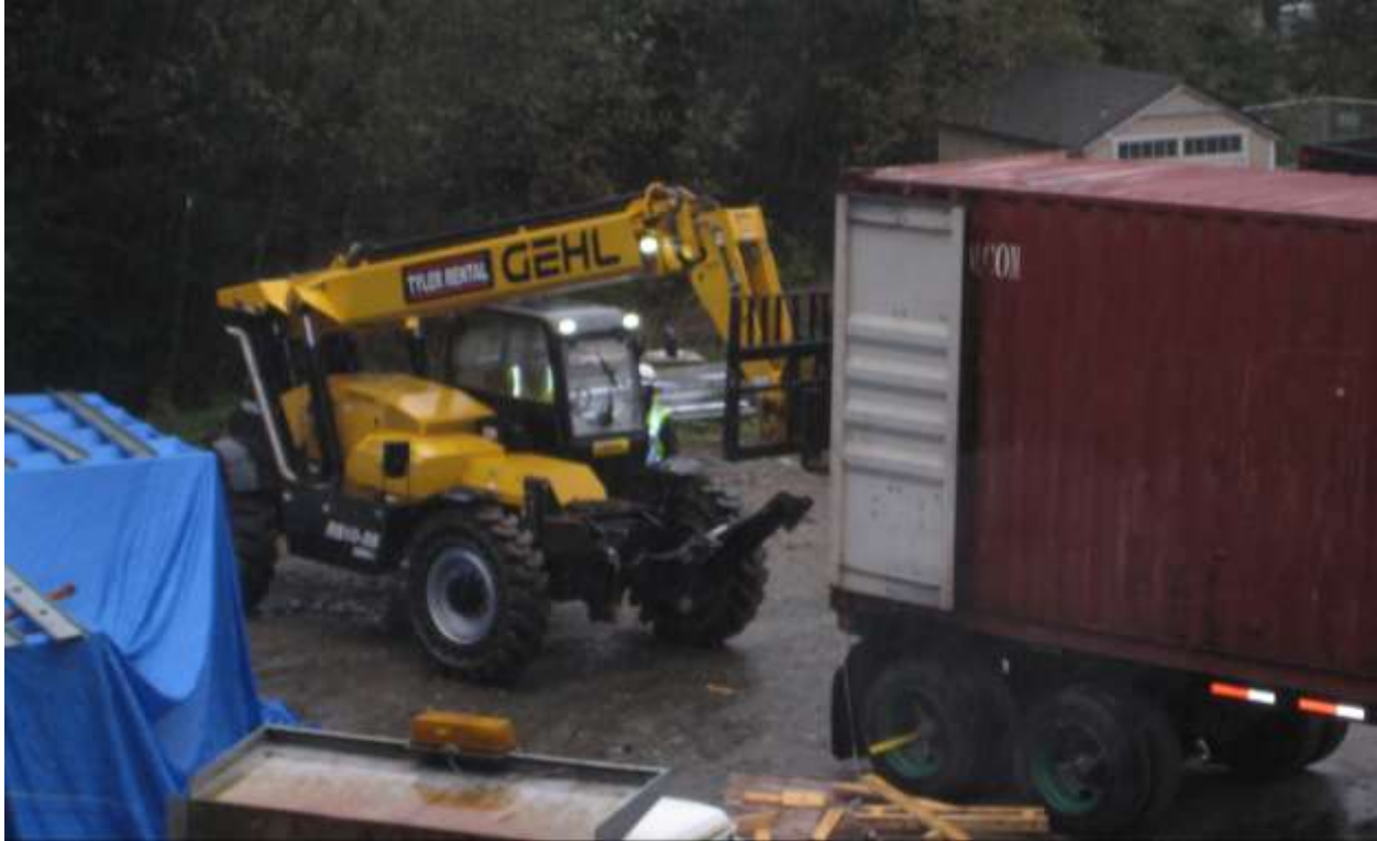
Photo 2679 – DC workers, Alex and Riley, offload elevator components from cargo container on the lower site level and transport them to the garage floor level.
