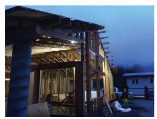
2. ACC had two workers continuing with asphalt shingle install over the north side of the south wing of the existing facility. ACC had two workers beginning on layout of offices starting with the north wall of Office 121 and Doctor 118. ACC had one more worker installing epoxy anchor bolts in plate on GL 7 per RFI 26.
