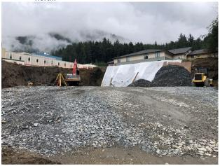
Concrete slab over existing 12" D.I. water line in path of excavation – subject of RFI #23.
