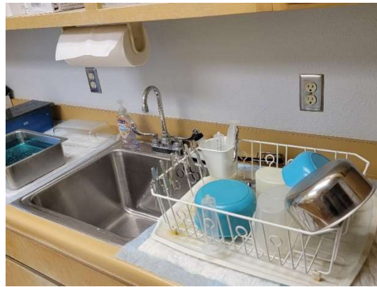
Outlets near sink
