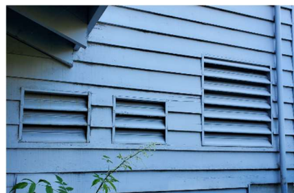
Boiler room relief and outside air louver
